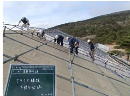
Fig. 2 Effect of reinforcement with aramid fiber A roof reinforced with the advanced fiber absorbed the impact when a fist-sized cinder crashed into it
